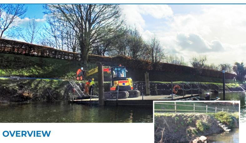
Steep marina banks were suffering from stability and erosion issues which, if left unchecked, would reduce their ability to withstand the wash of manoeuvring boats
